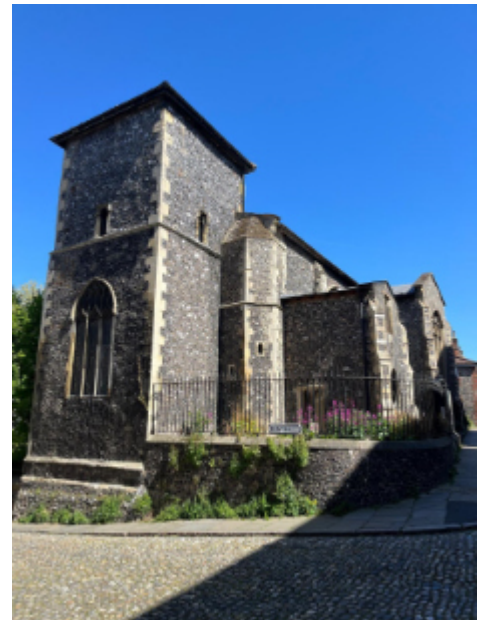
Right: church built with knapped flint walls
